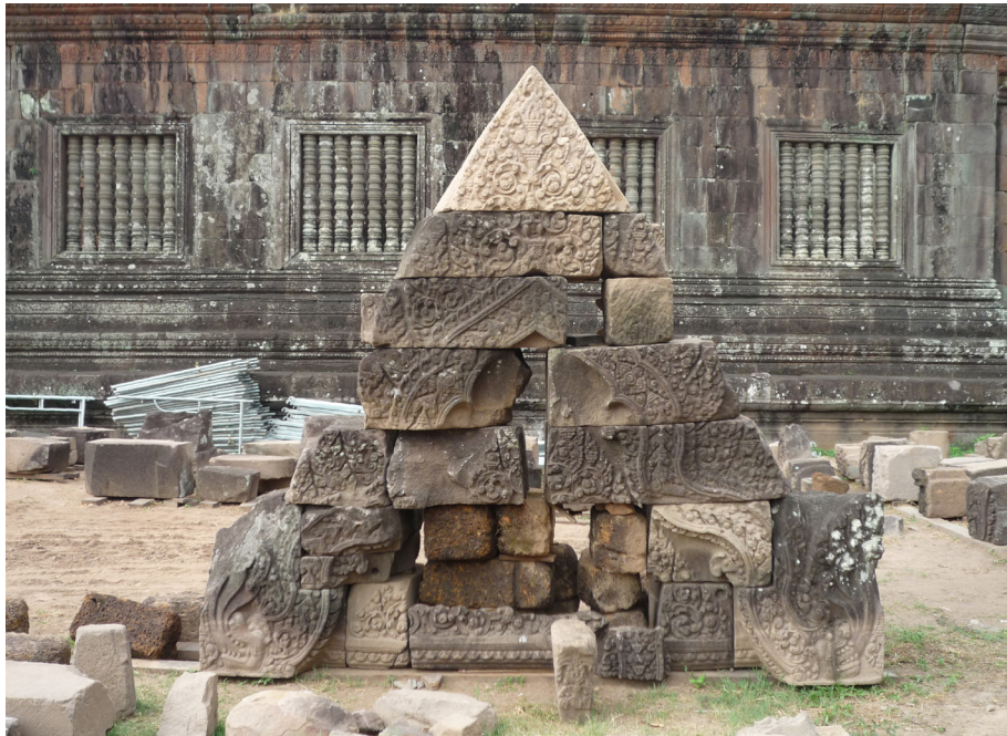
fig. 10 : Southern quadrangle gate, 2010. Sorting and recording recuperated blocks from the ruins for an initial reassembly before rebuilding the pediment. Missing stones will be replaced by new ones
