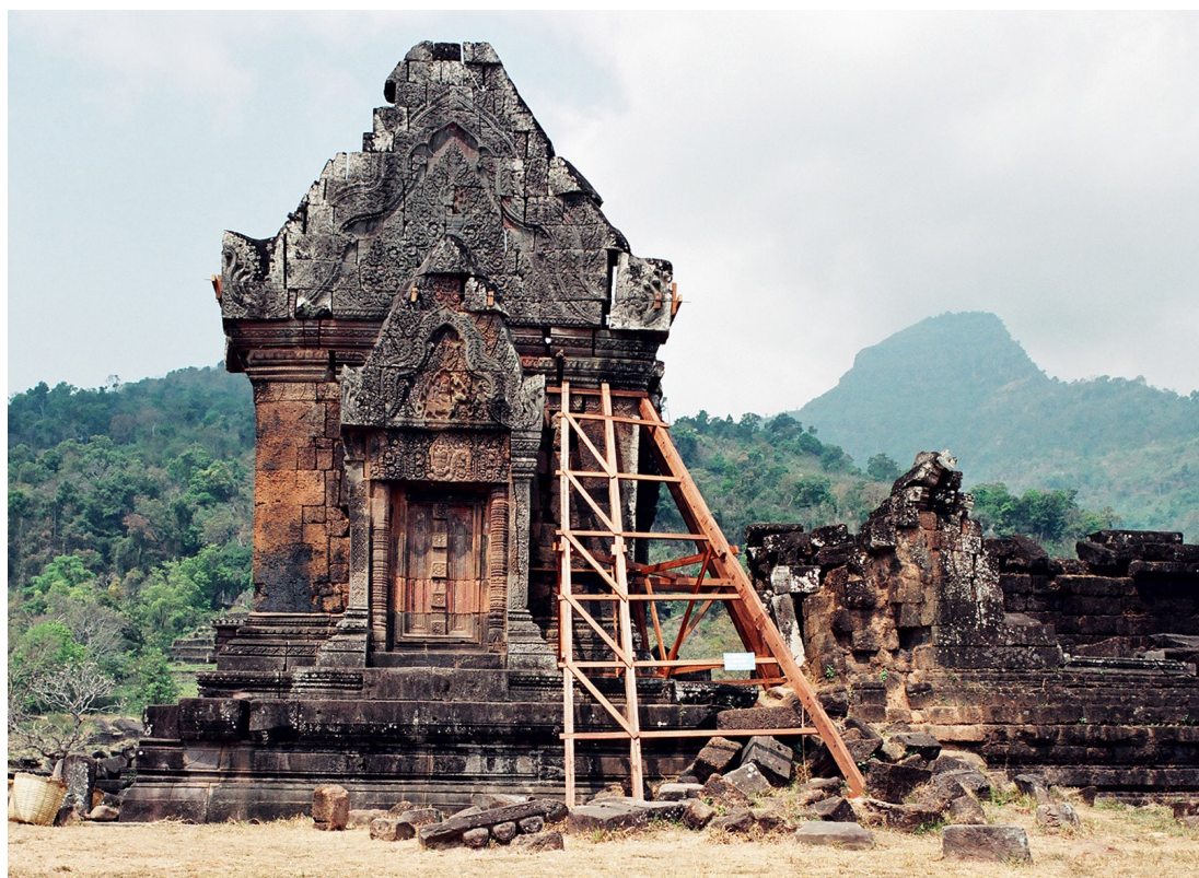
fig. 1: North quadrangle, 1997. Shoring up of a dangerously cracked angle in the main gallery
