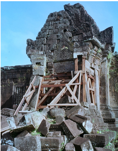
fig. 8 : North quadrangle, 2009. Supporting the entrance gate
