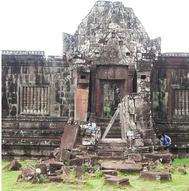
fig.7 : Entrance gate of the southern quadrangle, 2008. Fallen blocks obstruct the gate and the instability of superstructures makes this gallery off limits to the public
