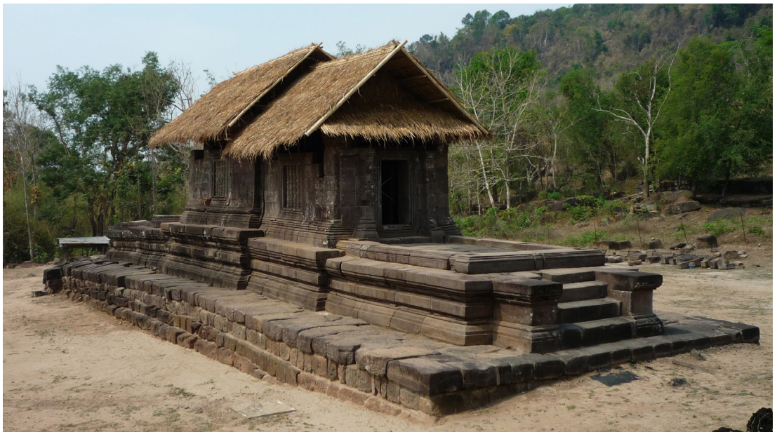
fig. 6: The southern building in 2010: in the forefront, the northern portion is rebuilt and stabilised. In anticipation of the rainy season, a temporary roof protects the central area where drains have not yet been installed
